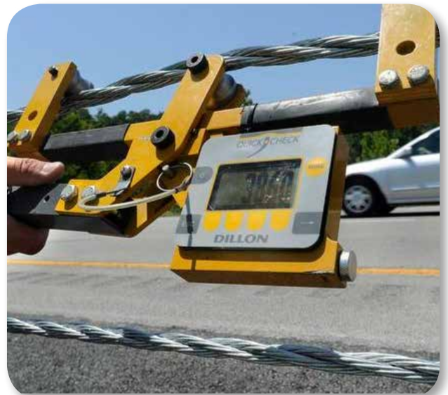
Measuring the cable tension
